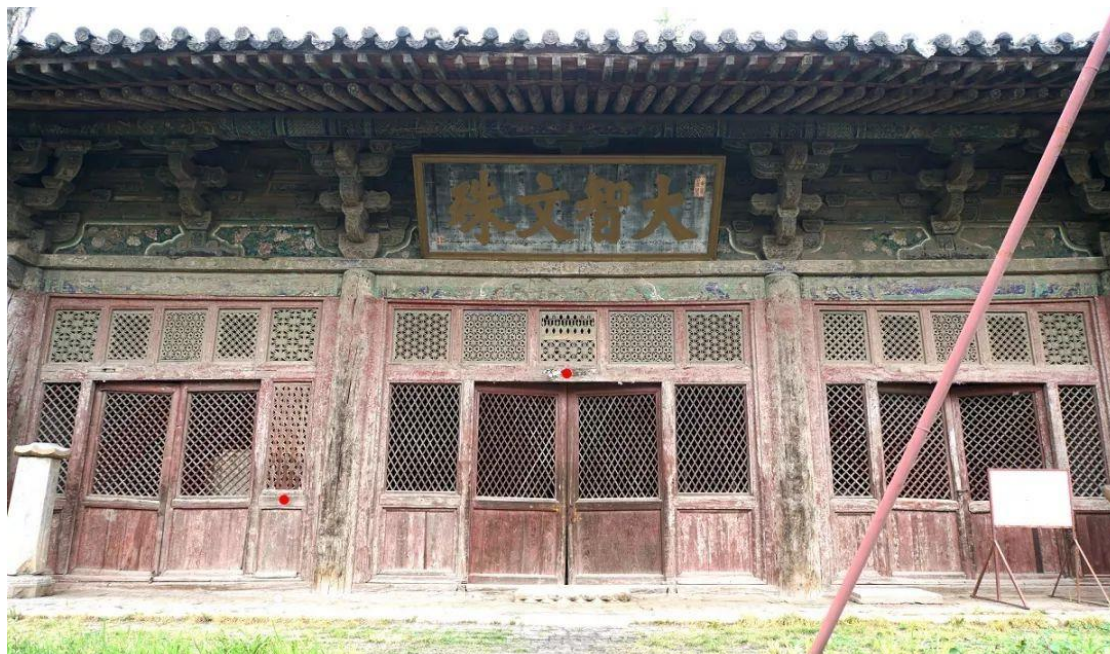
图6/阁院寺文殊殿正面门窗全貌
